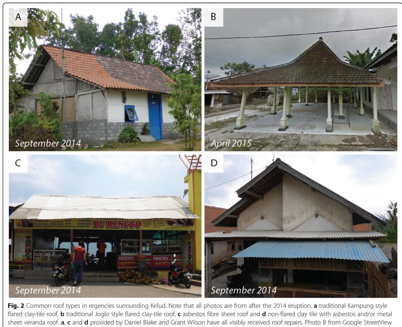
**Fig. 2** Common roof types in regencies surrounding Kelud. Note that all photos are from after the 2014 eruption. **a** traditional Kampung style flared clay-tile roof, **b** traditional Joglo style flared clay-tile roof, **c** asbestos fibre sheet roof and **d** non-flared clay tile with asbestos and/or metal sheet veranda roof. **a**, **c** and **d** provided by Daniel Blake and Grant Wilson have all visibly received roof repairs. Photo B from Google StreetView
