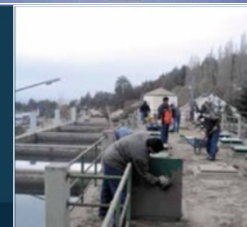
Ash can enter sand filter beds both from direct fallout, and through the intake. Cleaning of filter beds creates heavy additional labour demands, such as at Bariloche WTP following the June 2011 Puyehue Cordón-Caulle eruption (below)
