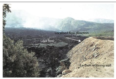
Fig. 2 Lava flow from the 1991–1993 eruption of Etna stalling behind an earthen barrier while an artificial channel is built downhill. Image modified from Barberi et al. (1993)
